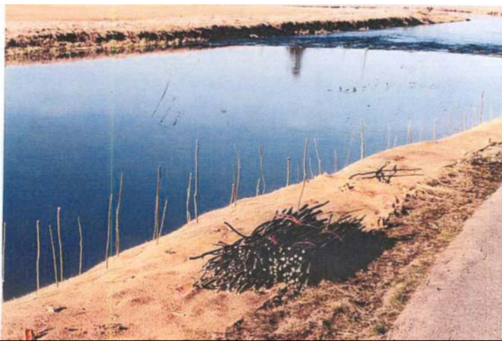
Willow cuttings were used hold and stabilize the bio-degradable jute fabric.
