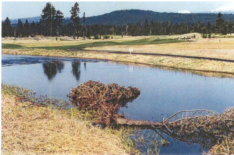
This late 1990's photo matches the introductory photograph in 2007. It shows the completed bank stabilization, dead trees in place, and a created riffle on the top left side.
